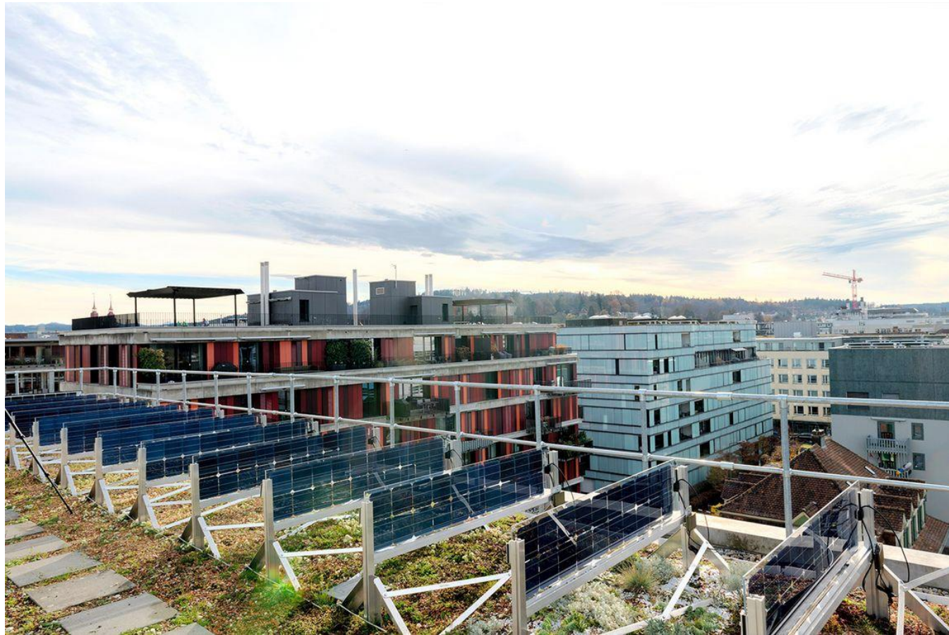
Vertical Bifacial Biosolar Green Roof
