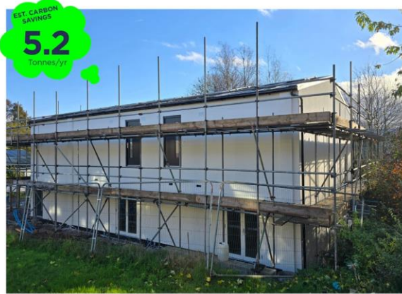
Crofts Estate 5 units (4 x 1bed, 1 x 2bed) Nearing Completion
